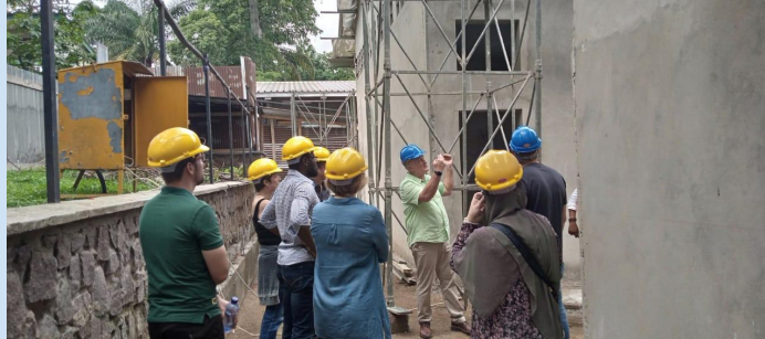
Current TASOK board members visiting the project site during their board retreat in November 2022
